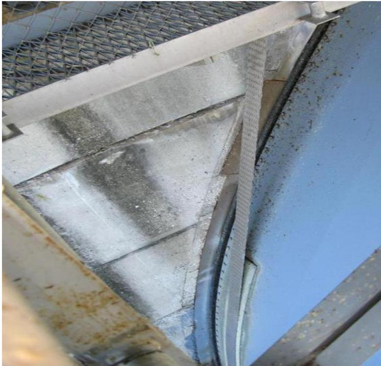
**Figure 1: Hoisting cable from Carlyle tainter gate. Picture from the experimental procedures performed by Dr. Gopalaratnam and Dr. Riveros in Carlyle Lake Dam.**
