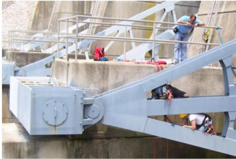
**Figure 30: Installation challenges. Picture from experimental procedures performed by Dr. Gopalaratnam and Dr. Riveros in Carlyle Lake Dam.**
