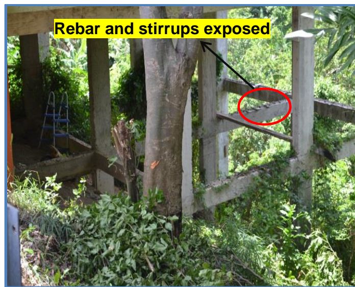
Figure 2-16. Residence with Exposed Rebar
