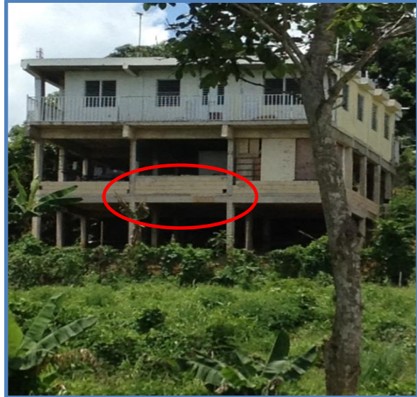
Figure 2-17. Residences with Vertical Irregularities
