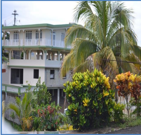
Figure 2-17. Residences with Vertical Irregularities
