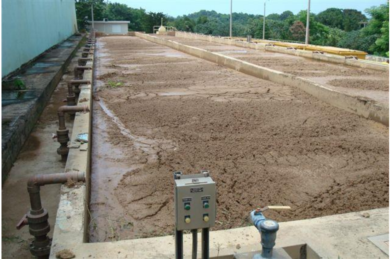
Figure 7. Miradero Water Treatment Plant Drying Beds
