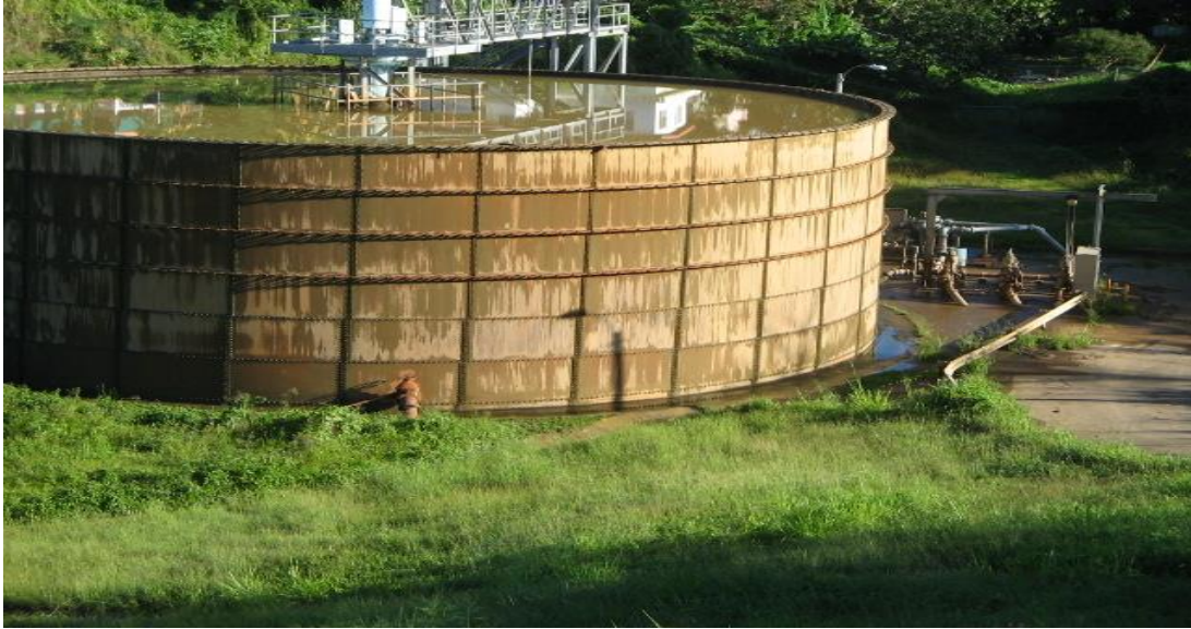
Figure 5. Miradero Water Treatment Plant Thickener
