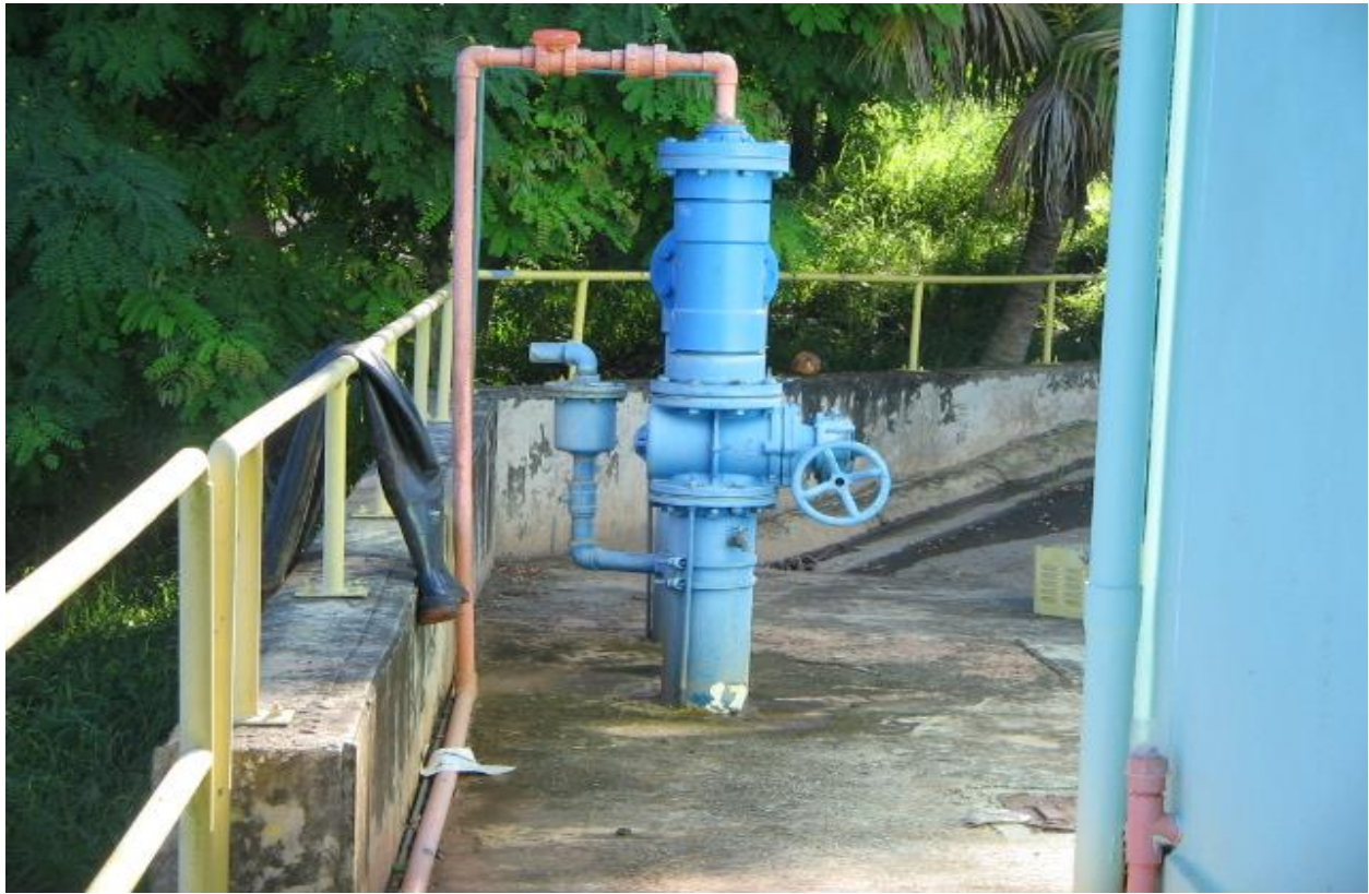
Figure 25. Sampling point #2 and polymer addition for suspended solid removal
