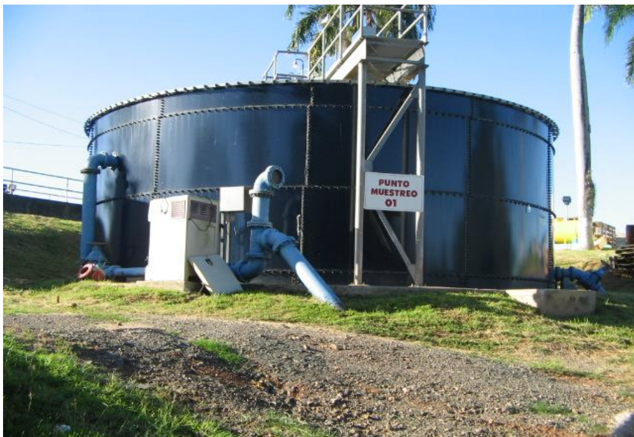
Figure 26. Thickener #2 and Discharge Point 001
