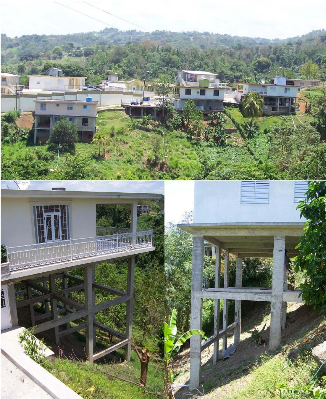
**Figure 1.1 - Examples of concrete frame structures supported on gravity columns in Puerto Rico**
