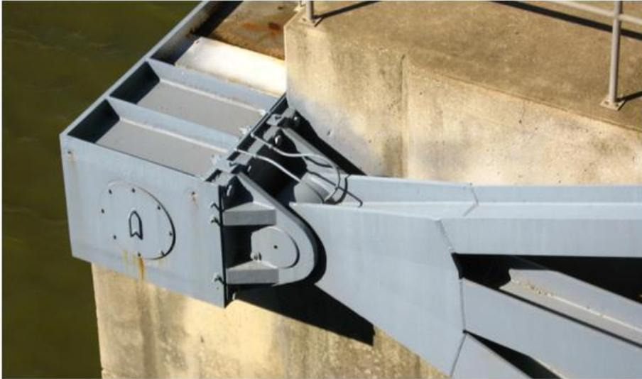
**Figure 13: Trunnion assembly of the Carlyle Tainter gate. Picture from experimental procedures performed in Carlyle Lake Dam by Dr. Gopalaratnam and Dr. Riveros.**
