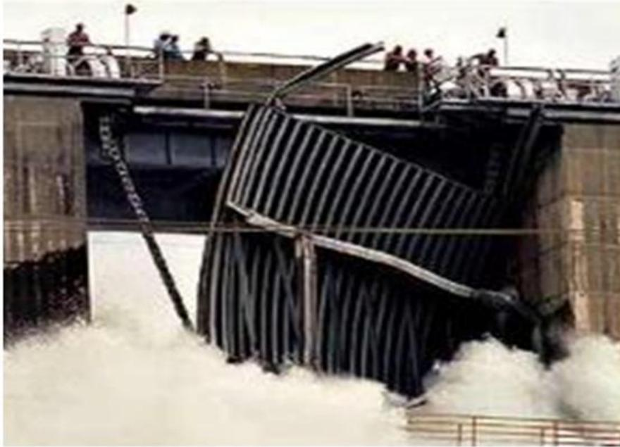
**Figure 5: Failure on tainter gate in Folsom Dam, CA. Picture from Forensic Report Spillway Gate 3 Failure Folsom Dam, Bureau of Reclamation Mid-Pacific Region, 1996.**
