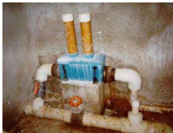
Figure A4-4: Photos of the Comunidad Aislada Unida en Desarrollo, Inc. water well; and the chlorination treatment system used in this water
