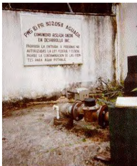
Figure A4-4: Photos of the Comunidad Aislada Unida en Desarrollo, Inc. water well; and the chlorination treatment system used in this water
