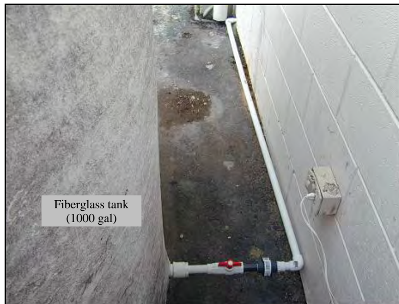
Figure 3-3: Plumbing System outside the Environmental Engineering Laboratory
