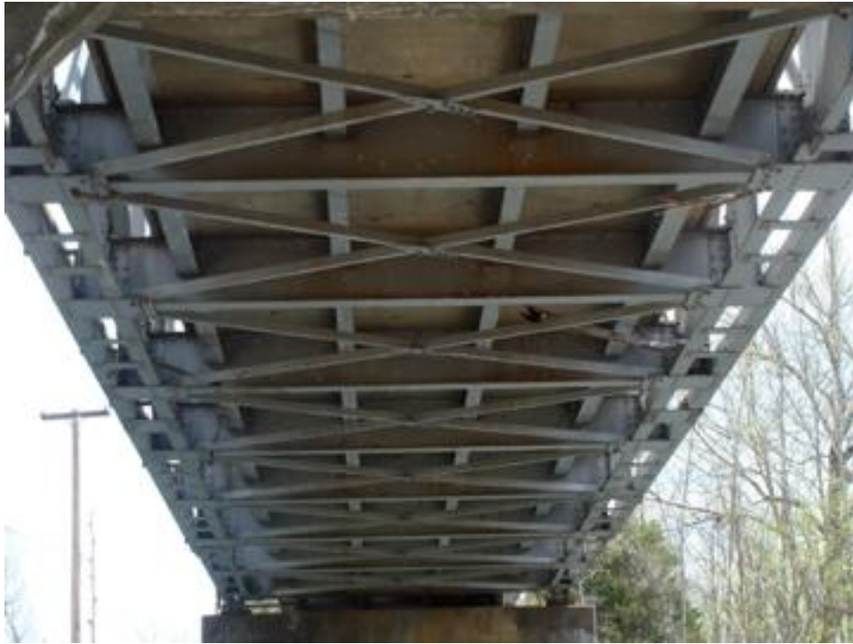
FIGURE 8: PLAN VIEW OF STEEL TRUSS BRIDGE SPAN.
