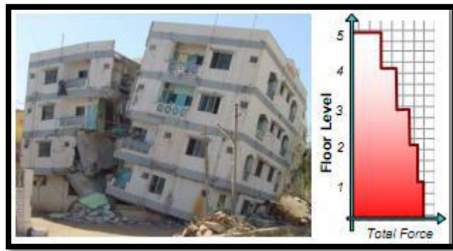
Figure 1-1: Total Horizontal earthquake forces in a building increase downward along its height.
