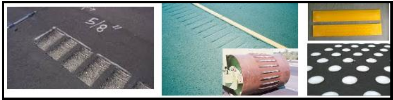
Figure 2.3 Milled in, Rolled or Raised Rumble Strips (Google Images, 2014)
