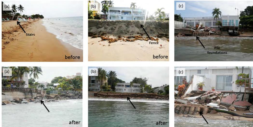
**Figure 1.7:** Extreme erosion at the coast of Rincón caused by tropical storm Isaac. The photos identified by the same letter represent the same location (from Chardón, 2013).
