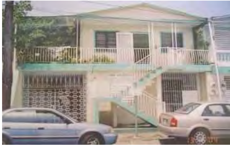
Figure 11.6 - Second story all-wood residential addition
