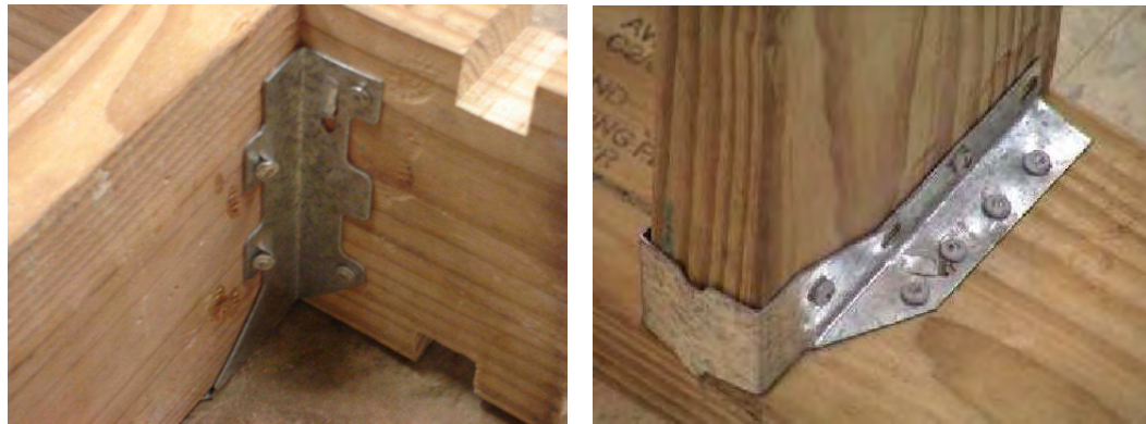
Figure 4.1 - Variable connectors between joist and rafter
