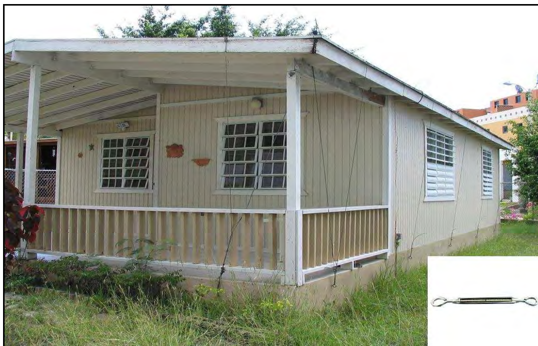
Figure 7.11 – Picture of guy implementation and turnbuckle
