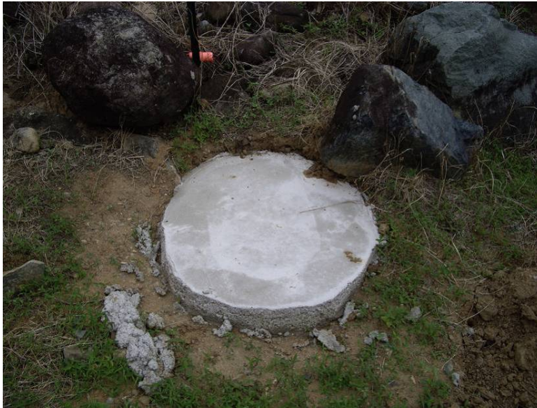
Figure 3-3. Example of Concrete Pad for Sensors on Slope
