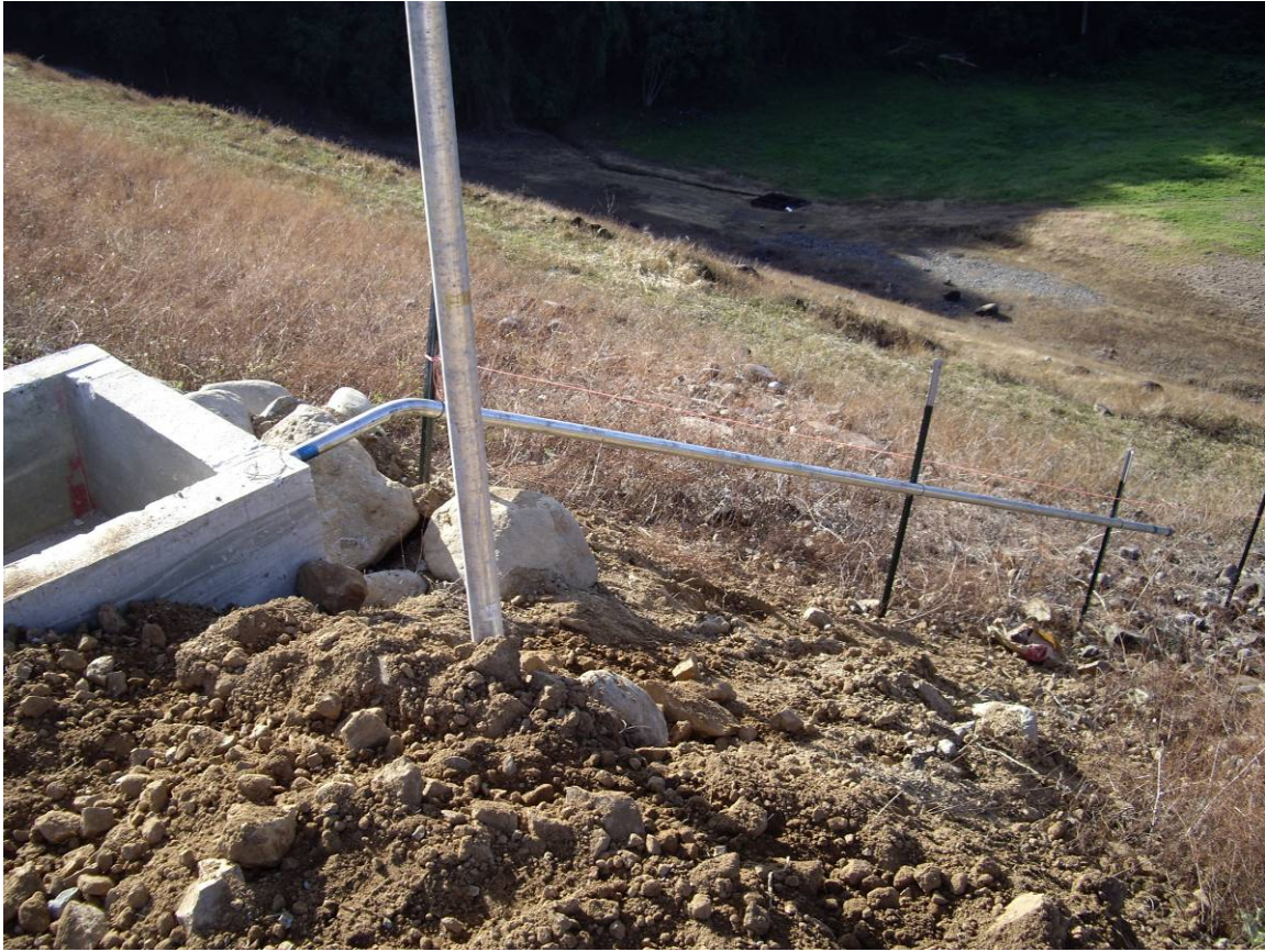
Figure 3-6. Example of Exposed Piping Used in Patillas Dam
