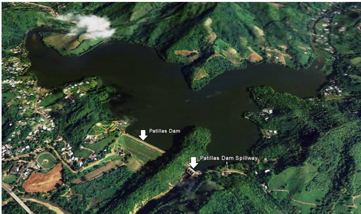
Figure 2-6. Aerial View of Patillas Dam and Spillway
