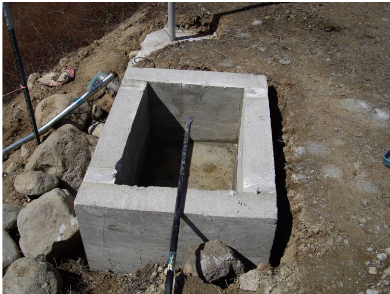
Figure 3-4. Concrete Box for Digital Recorders at the Crest
