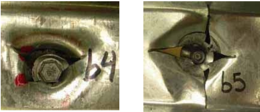
Figure 32 Failure of Screwed connections by García, 2008, pp. 65.
