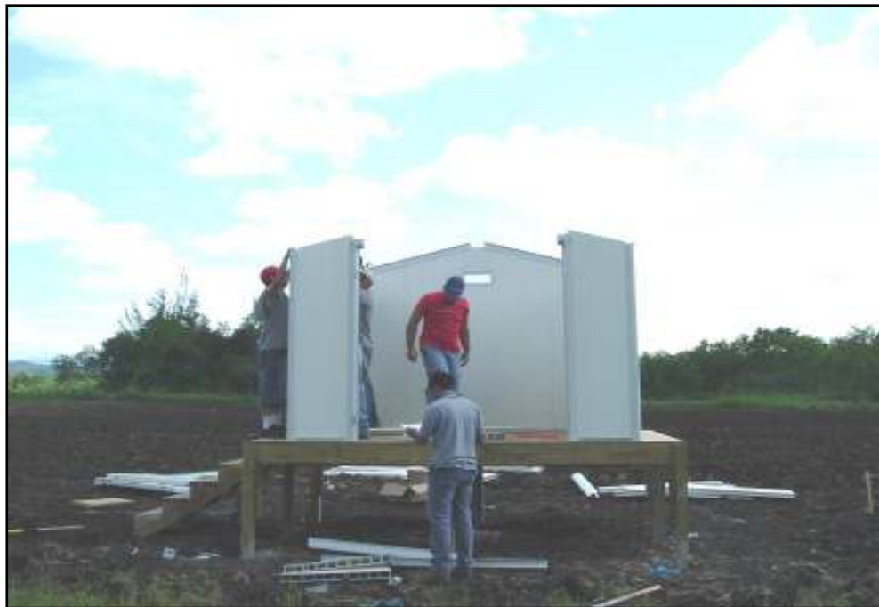
Figure A5. Shed Installation
