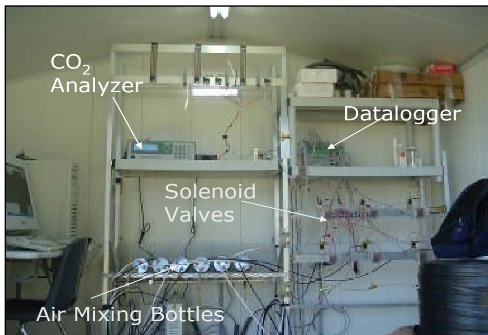
Figure B3. Instruments inside shed for monitoring chambers and ambient plots.
