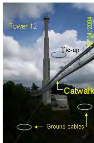
Figure 1.9. Catwalk (pedestrian bridge) and supporting cables (photo by author)
