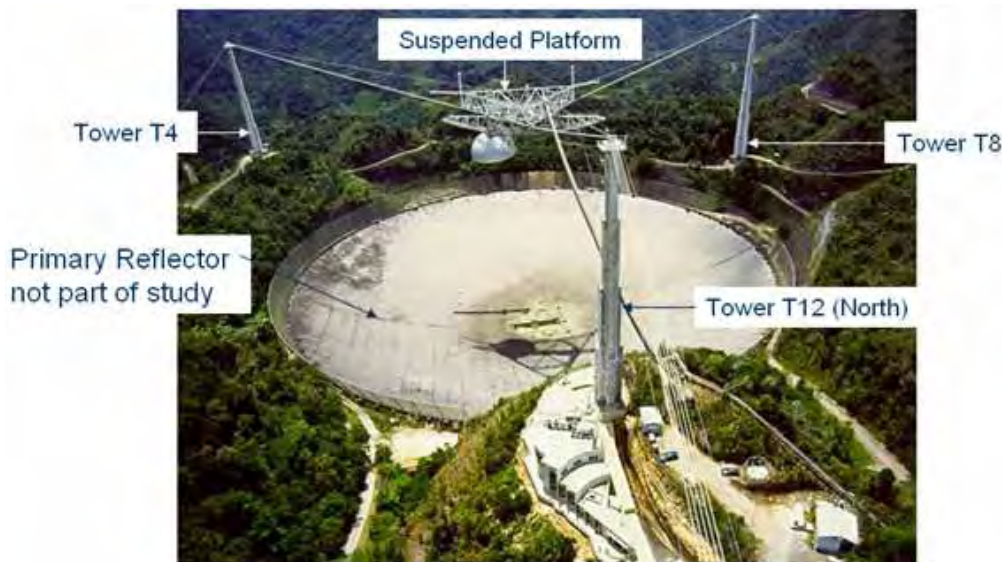
Figure 1.1. Overall view of the Arecibo Observatory (courtesy of NAIC)
