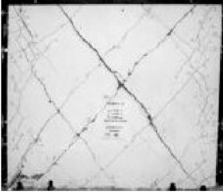
a) Diagonal tension failure of wall 27 tested by Hidalgo et al. (2001)
