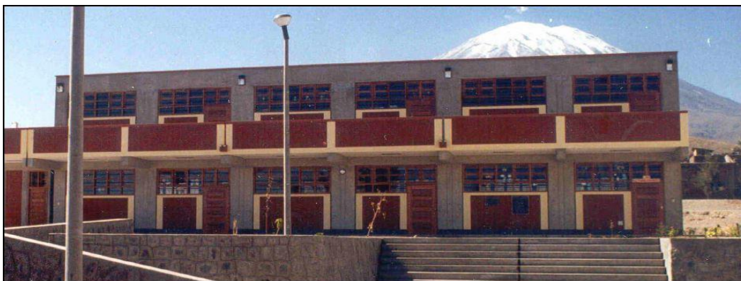
Figure 19. Modern school building, after 1997, undamaged in the Atico earthquake, Peru, 2001.
