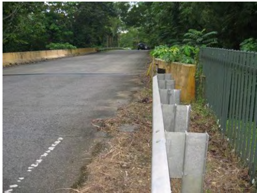
Figure 37. Eastbound Entry Transition of Bridge #2231
