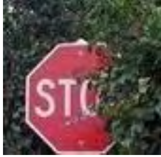
Figure 28. STOP Sign Partially Covered by Foliage
