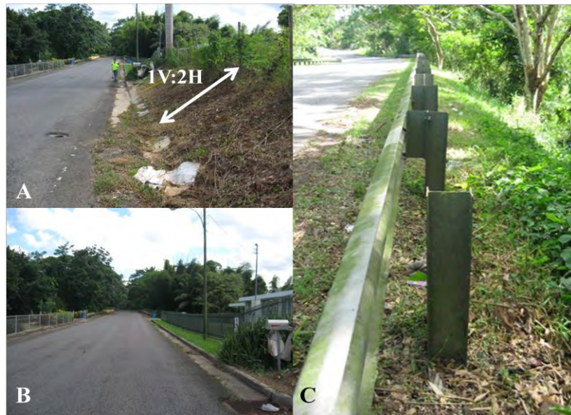
Figure 35. Issues Encountered on Bridge #2231 Eastbound Approach
