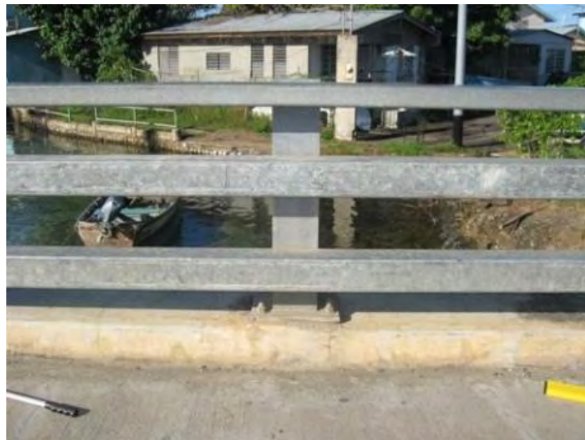
Figure 40. Bridge Railing 3 Tube Curb Mount
