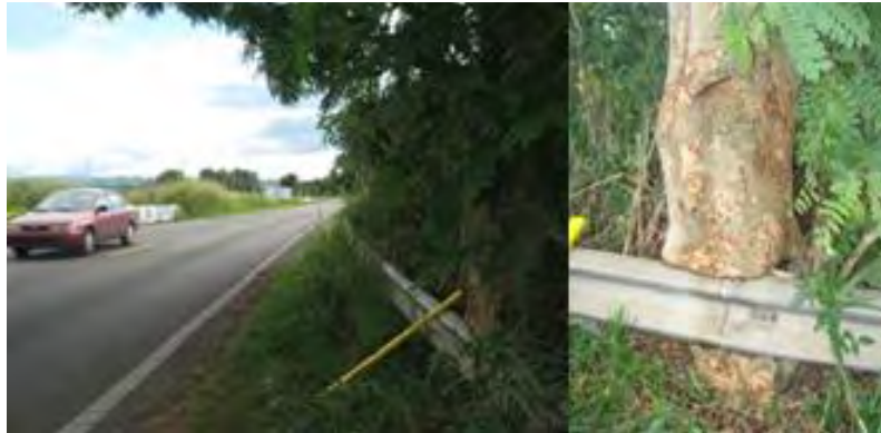
Figure 33. Tree Behind Approach Guardrail
