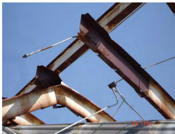
Figure 8.22: Case #1, close up photograph of roof beams showing buckling and extreme corrosion damage.
