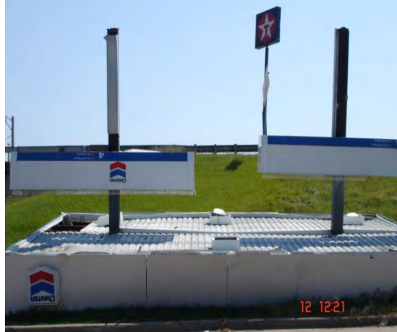
Figure 8.39: Case #3, additional photograph of the inverted steel structure.
