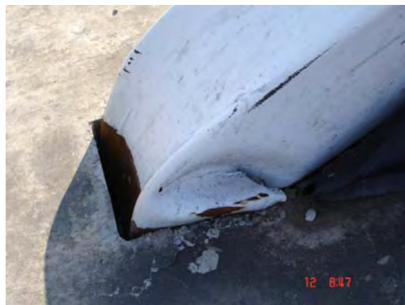
Figure 8.44: Case #4, photograph showing closer detail of the buckled steel columns.
