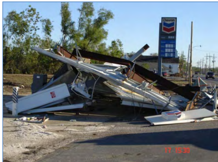
Figure 1.4: Canopy structure collapsed at Meraux, New Orleans, Hurricane Katrina, (Photograph by L. Godoy).
