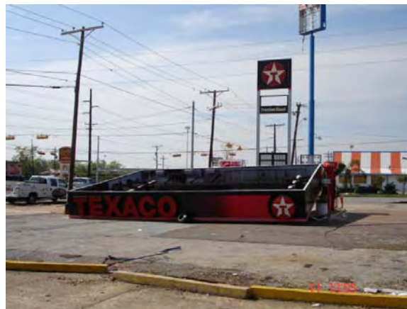
Figure 8.27: Case #2, open canopy structure completely collapsed.
