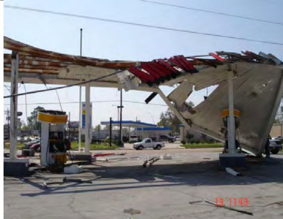
Figure 8.21: Case #1 transversal view of the deformed and collapsed roof.
