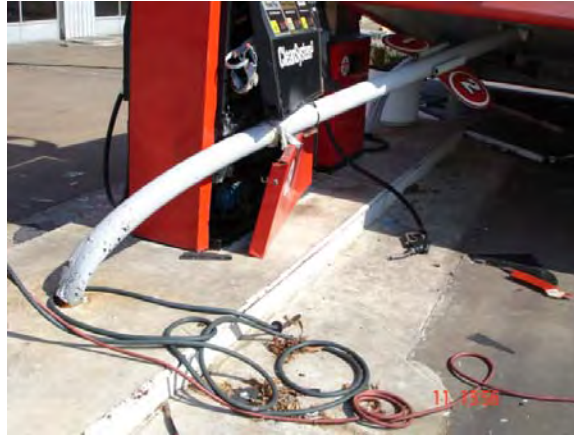
Figure 8.28: Case #2, photograph showing a buckled round steel column.
