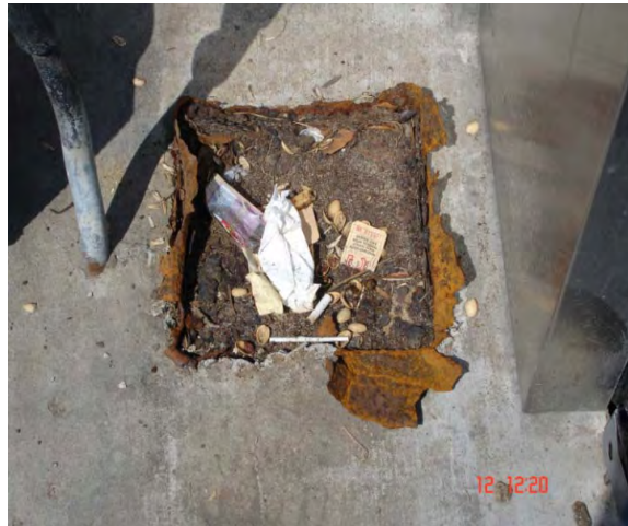
Figure 8.38: Case #3, photograph of the existing corrosion condition at the column base.
