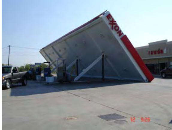
Figure 8.45: Case #4, photograph showing the collapsed steel columns.
