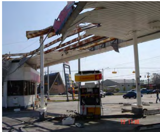
Figure 8.19: Case #1 partial collapsed roof from below. Bottom of roof cladding has been taken away due to high wind pressures.
