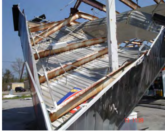
Figure 8.18: Case #1 collapsed roof layout showing some of the roof beams damages. Permanent deformation is clearly shown on some of the roof members.
