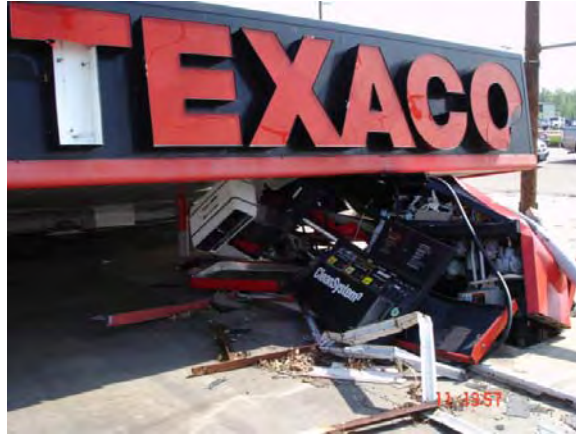
Figure 8.30: Case #2, photograph showing the open canopy structure on top of the gas pumps.
