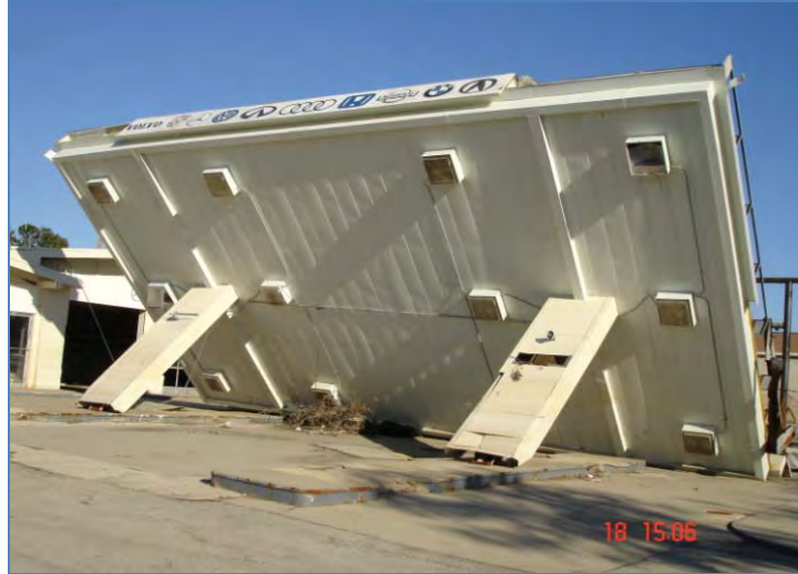
Figure 1.3: Failed canopy in Chalmette, New Orleans, during Hurricane Katrina, (Photograph by L. Godoy).
