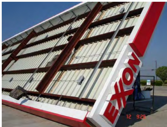
Figure 8.46: Case #4, additional photograph of buckled steel columns. The photograph shows the internal column flange.
