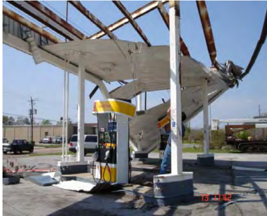
Figure 8.20: Case #1 roof cladding and beam structural layout. Photograph showing permanent deformation on roof members.
