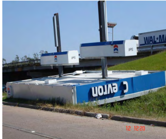
Figure 8.37: Case #3, open canopy photograph of the inverted steel structure after the steel columns failed due to corrosion and wind pressures.
