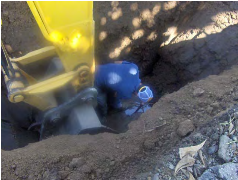
Figure 4.2 Sampling excavation pit
