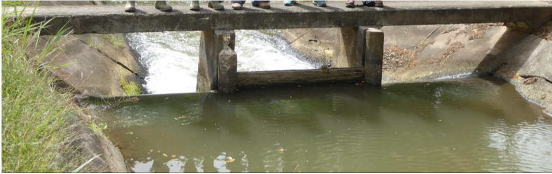
Figure 5.13. Inline weir located at the main channel downstream from the junction between the main channel and the lateral channel M63 at the Lajas Valley Irrigation District System.
