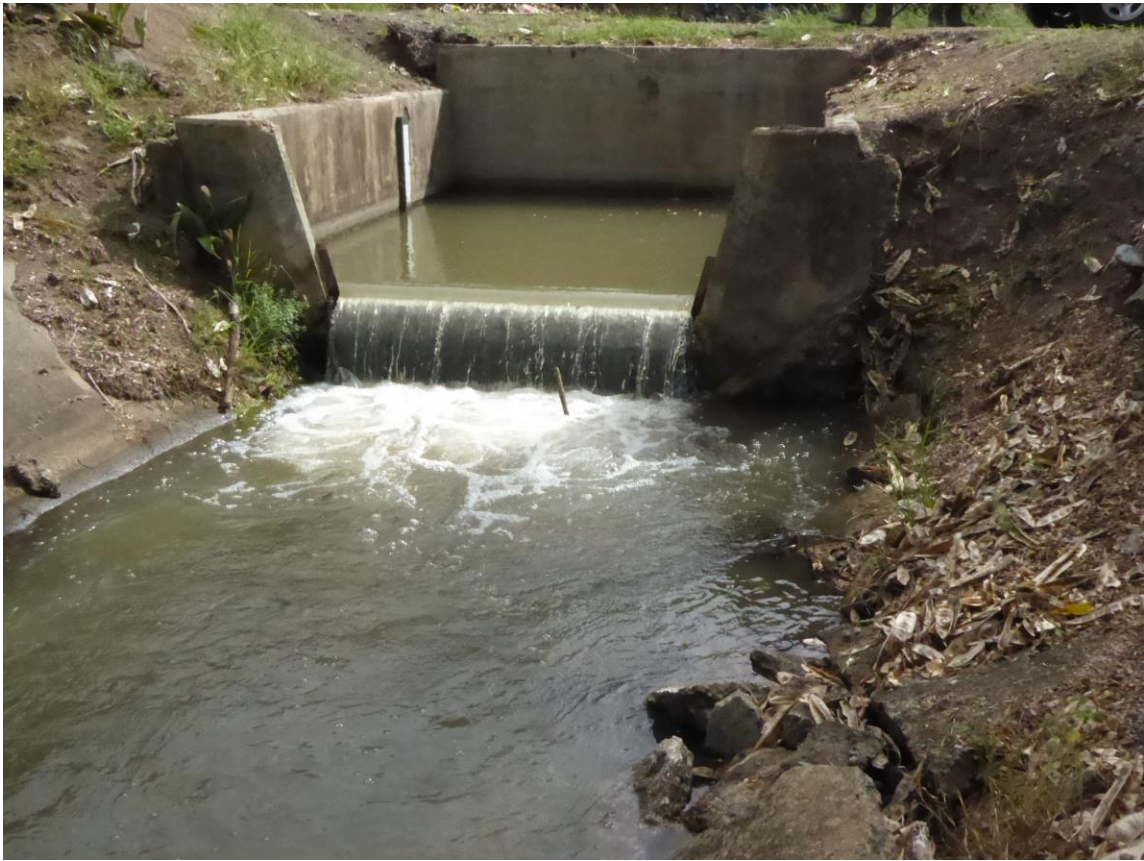
Figure 5.14. Stilling basin and trapezoidal weir located at lateral channel M-63 at the Lajas Valley Irrigation District System.
