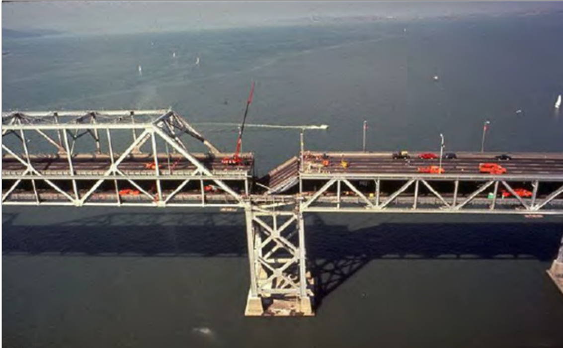
Figure 1. 2. Damaged bridge in San Francisco, CA: Loma Prieta earthquake, (FHWA 2011).
