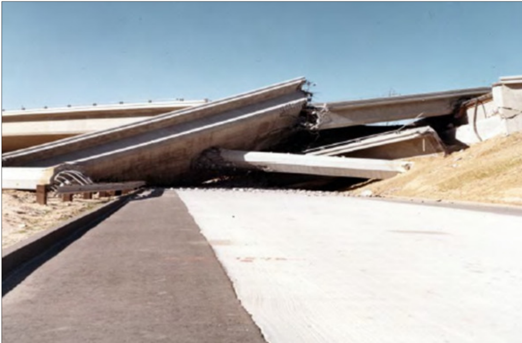
Figure 1. 1. Collapsed bridge in I-5, SR-14 Overpass: San Fernando earthquake (FHWA 2011).
