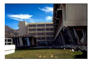
Figure 1-1 Olive View Hospital, San Fernando, California, after the 1971 San Fernando Earthquake. [Adapted from www.cartage.org]
