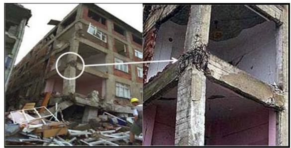
Figure 1-2 Collapse due to beam-column joint failure [Adapted from Pantelides et al. 2002].
