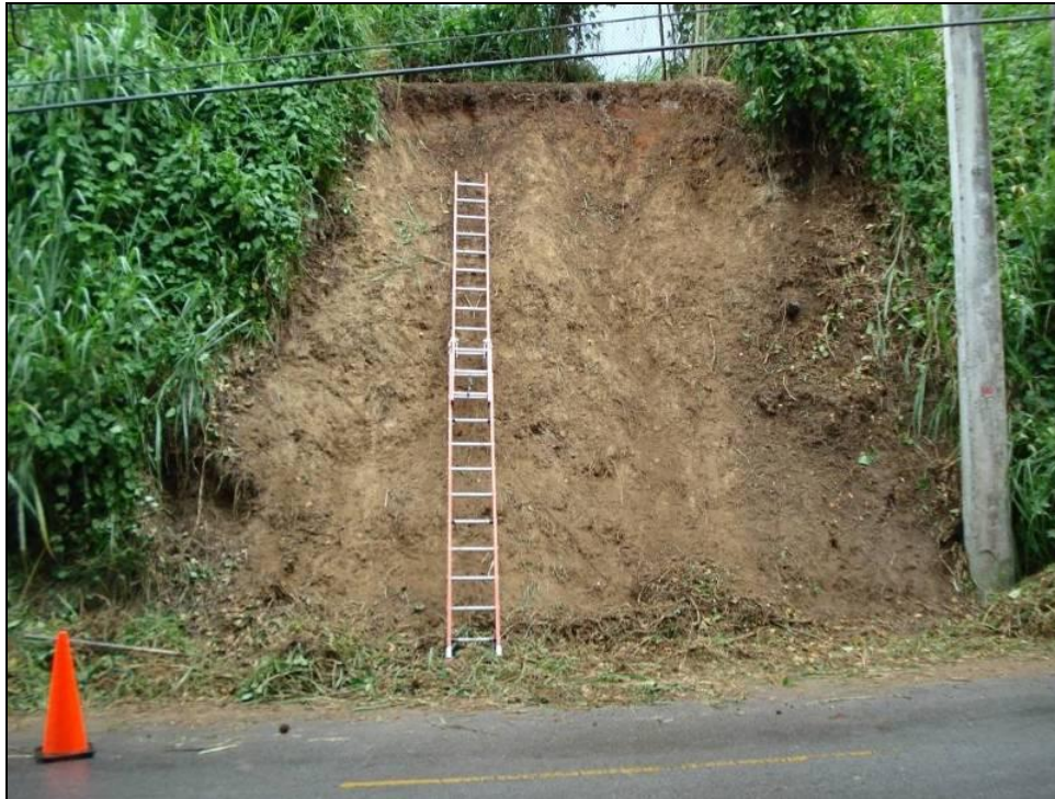
Figure 5.6 Slope cleared of vegetation for instrumentation.
