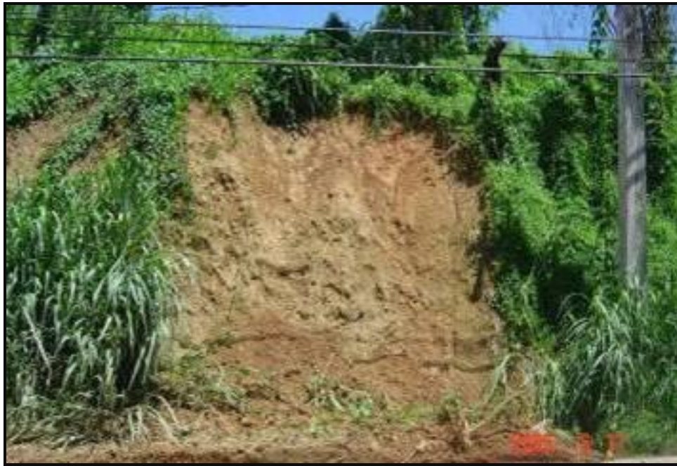
Figure 4.8 Slope under study one week after failure.
