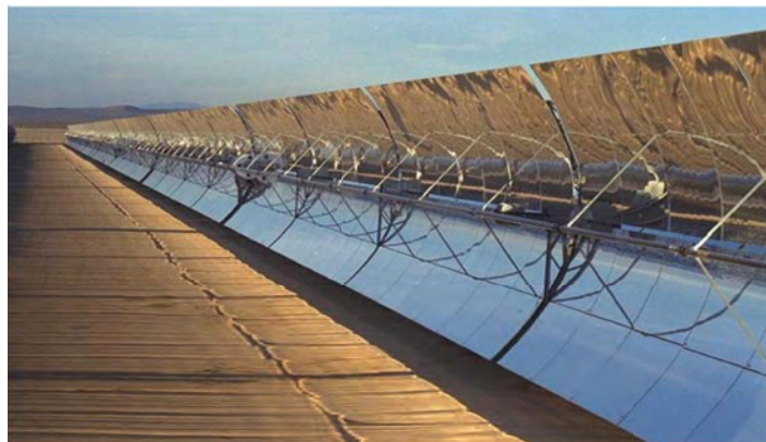
Figure 4.3: Collectors and absorber in a parabolic trough plant (NREL)
