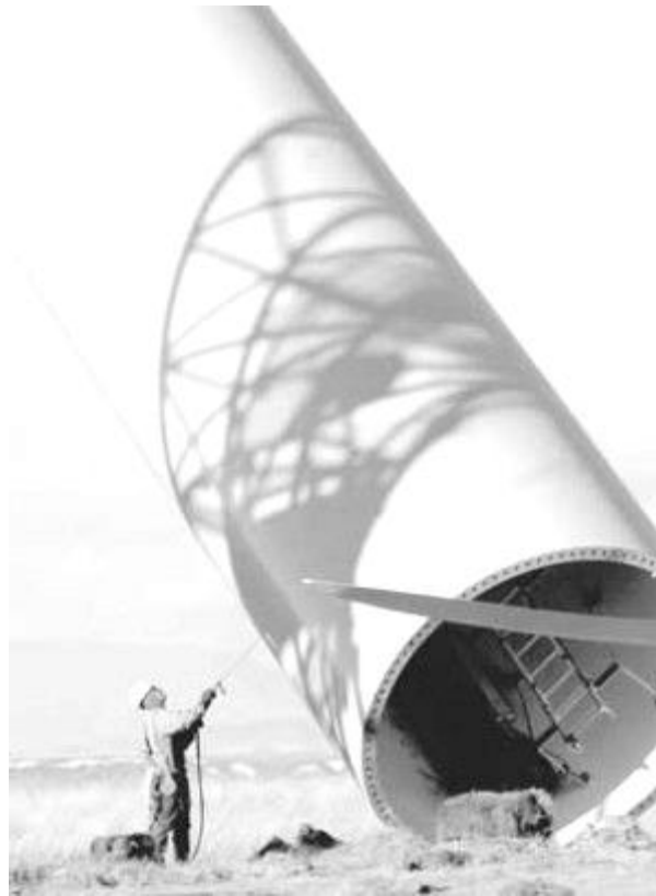
Fig. 1-4: The first tower section is hoisted into position (from Billings Gazette, n.d.)
